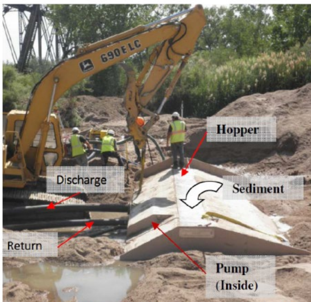
Figure 3. Components of the Sediment Collector™ at the Fountain Creek, CO Install (Tucker et al., 2015)
